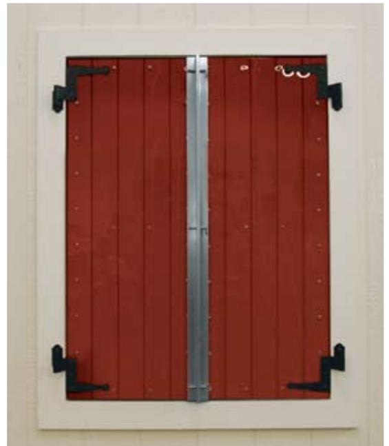
Board and Batten shutters closed with vertical storm bar system.
