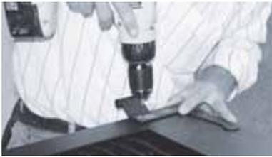
2. Install hinges after determining offset. Hinges are to be set at top and bottom even with outside. Drill holes with 1/8th pilot bit. Be careful not to drill all the way through shutter.
