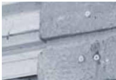
6. Install acorn clip. Swing shutter open and mark center of holdback clip and install acorn clip into brick.
