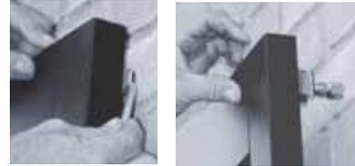
7. Install "S" Holdback\*. Shutter is now held open by acorn anchor. Position shutter dog in correct location and mark for screws and fasten to wall—1 1/2" down from shutter
