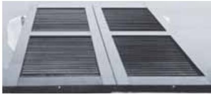
1. Pick shutters to fit window and put next to each window on top of saw horses to make sure shutters are paired properly. Lay two shutters face down next to each and prepare to install hinges.
