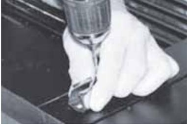
3. Position and install upper holdback clips 1" from top and center edge of stile. Shutters over 58" require 2 sets of acorns; install similarly at top.
